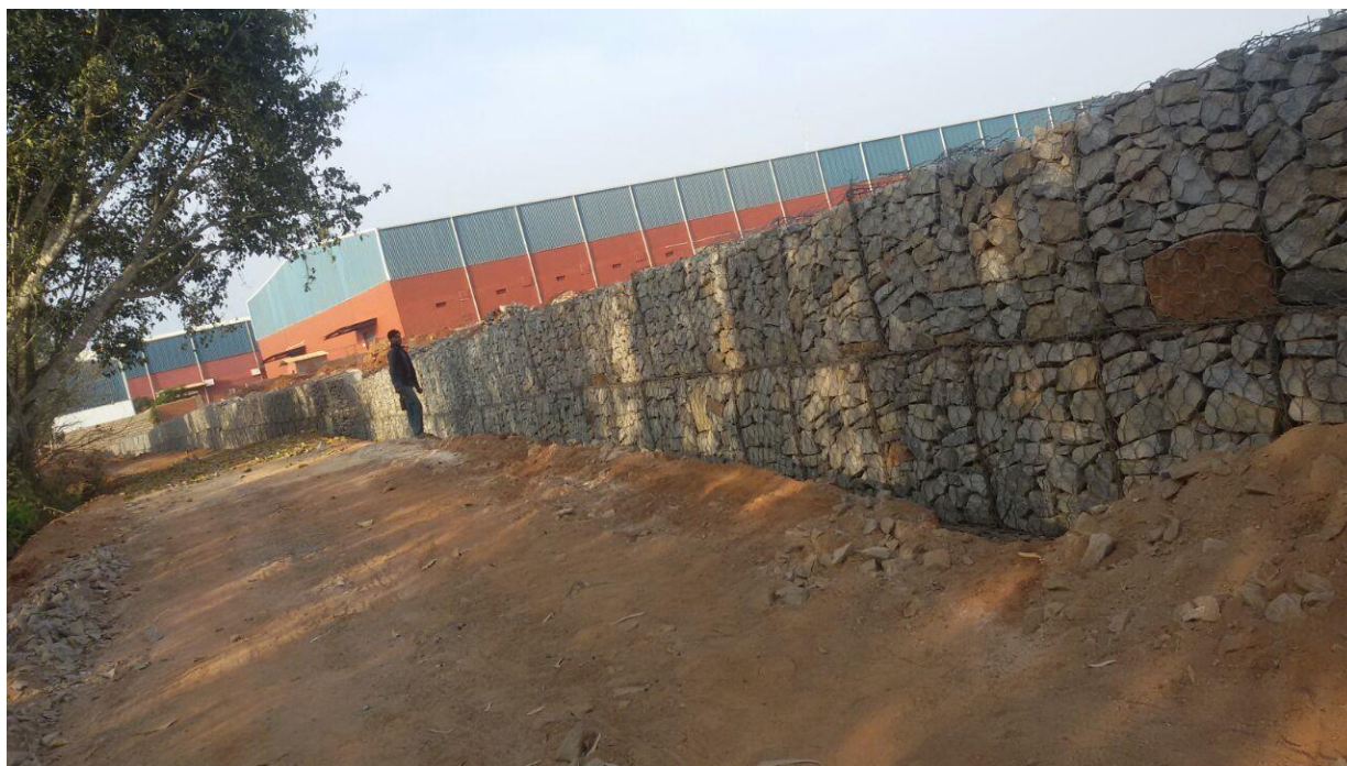
2 meter height Gabion wall
