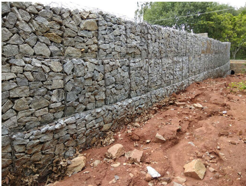
2 meter height Gabion wall
